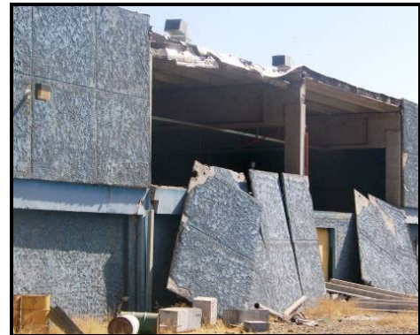
Precast reinforced concrete construction at Ciudad Empresarial. Inadequate wall panel connections resulted in building damage.
