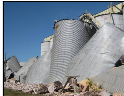
Collapsed thin-walled steel grain tanks.
