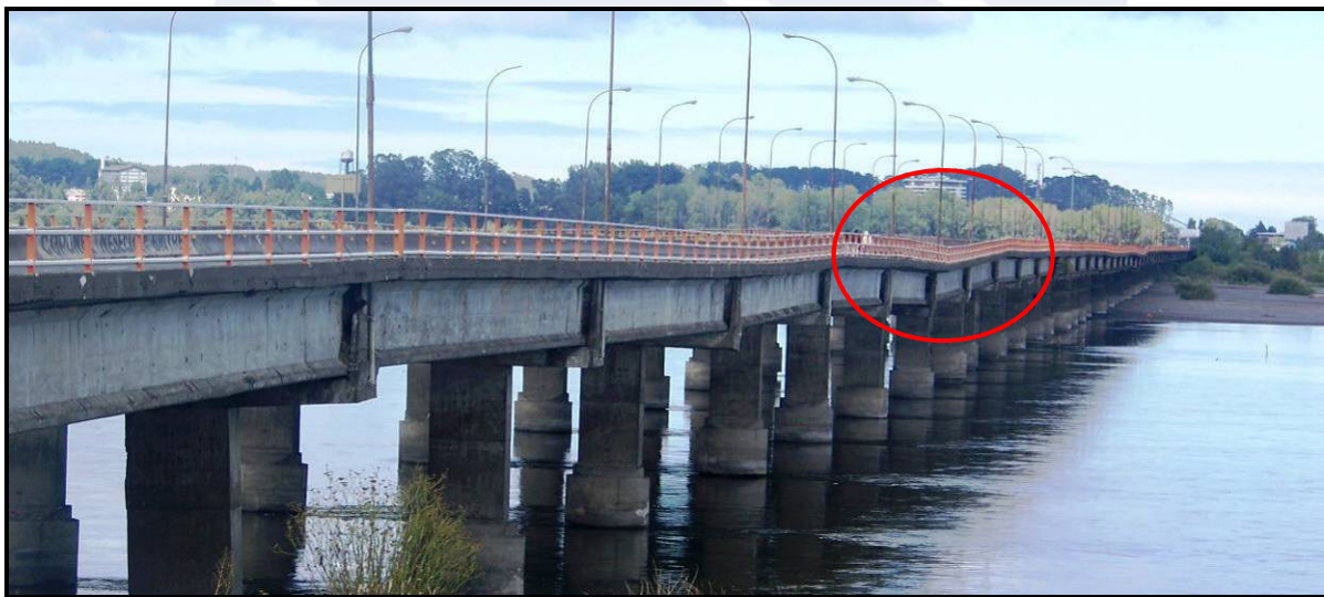
Juan Pablo II Bridge damaged in the February earthquake was restored to service in October 2010. This photo from March 2010 illustrates some of the bridge foundation damage as evidenced by the sagging roadway.
