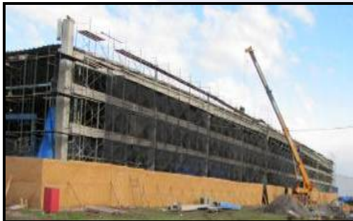
Repairs at a production plant (Lampa)
