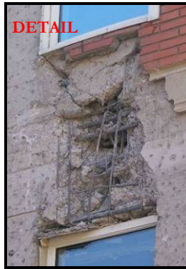
Example of extensive structural damage at Ciudad Empresarial (Santiago area). This recent vintage five-story office building suffered extensive damage (see detail). Irregular layout and weak soils contributed to the damage.
