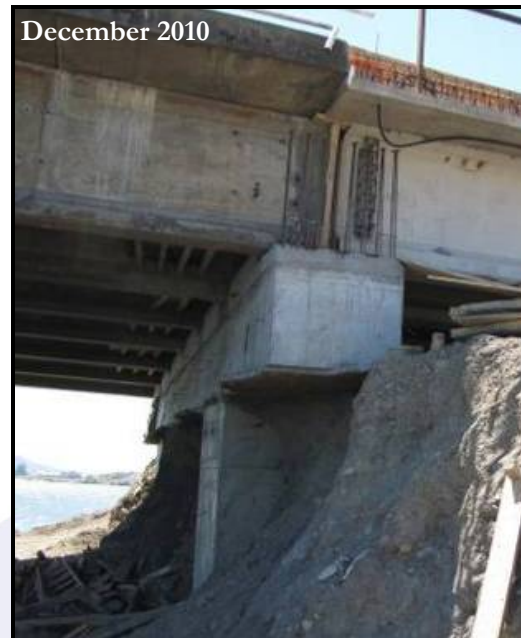
The photo on the left shows Juan Pablo II Bridge fractured column caused by soil liquefaction and lateral spreading along the the Bío Bío riverbank. The photo on the right depicts the new bridge girder and columns.
