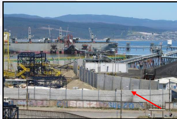
Tsunami-prone areas of Port of Coronel (south of Concepción) are surrounded by new flood walls.
