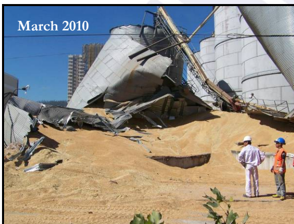
Concepción City Center: Collapsed grain bins have been removed but not yet replaced as shown in these two images taken in March and December of 2010. The 20-story residential tower in the background remains vacant. The right photograph includes the toppled Rio Alto tower (circled) which is still under investigation.
