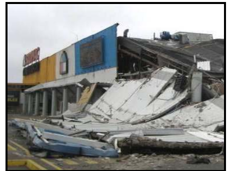
Collapsed concrete tilt-up wall panels due to weak wall-to-roof connections.
