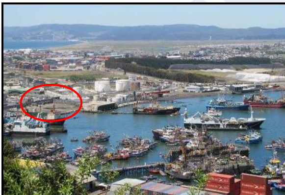
San Vicente Bay's industrial zone is recovering. A fish-processing plant (circled) has been demolished. Beach area was contaminated due to broken petroleum lines.
