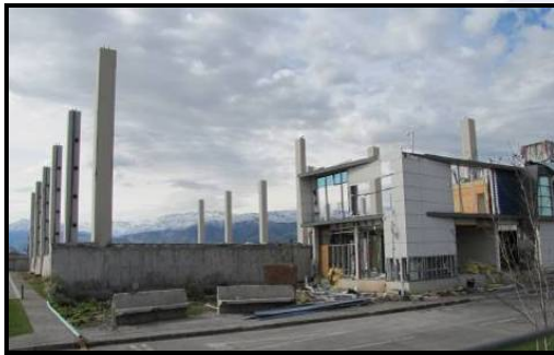
Destroyed modern industrial facility (Lampa)
