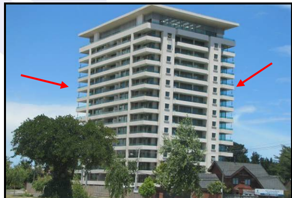
Damaged condominium tower in San Pedro still stands vacant. Corner balconies remain shored up.
