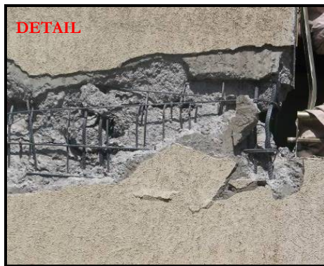
Modern high-rise residential tower in Santiago with extensive reinforced shear wall damage, as shown on the close-up photo. This building could not be occupied for months.
