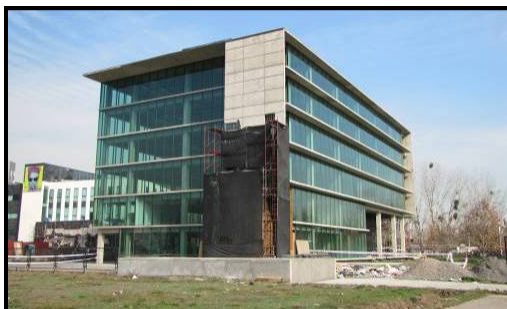
Office building repairs (Ciudad Empresarial)
