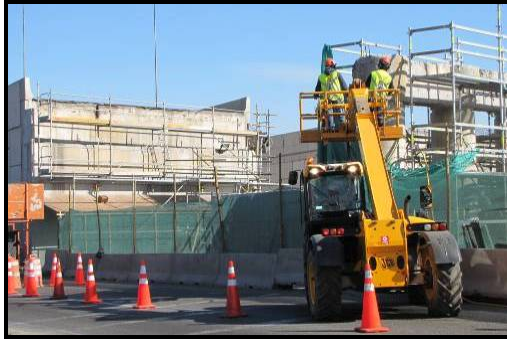
Collapsed bridge repairs (Vespucio Norte Highway)
