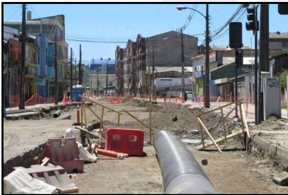
Street and utility reconstruction in Talcahuano city center is evident throughout the low-lying areas of this community.
