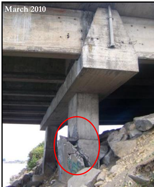
The photo on the left shows Juan Pablo II Bridge fractured column caused by soil liquefaction and lateral spreading along the the Bío Bío riverbank. The photo on the right depicts the new bridge girder and columns.
