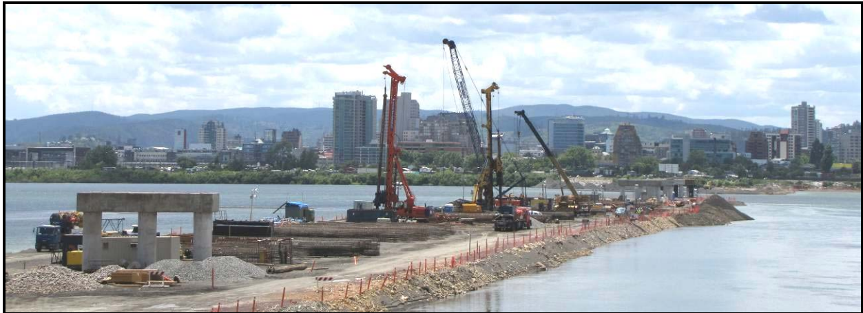
December 2010: Construction is in progress on a new highway bridge over the Bío Bío River in Concepción. This crossing will replace a bridge damaged by the earthquake. The city skyline (background) includes a number of vacant residential towers.
