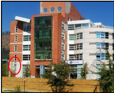
Example of extensive structural damage at Ciudad Empresarial (Santiago area). This recent vintage five-story office building suffered extensive damage (see detail). Irregular layout and weak soils contributed to the damage.
